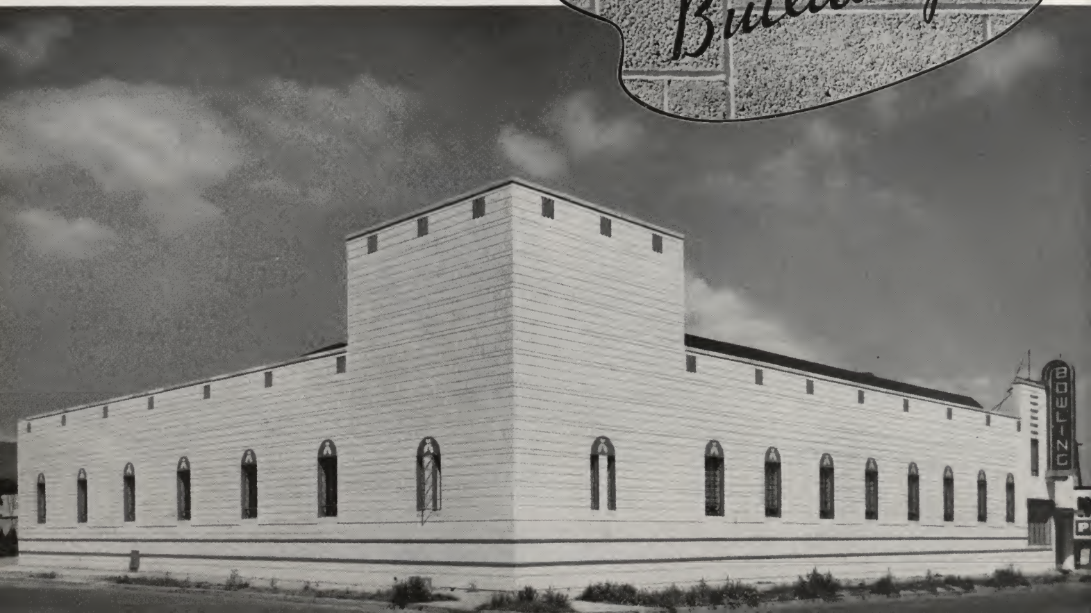
Below —Concrete masonry was used for both the exterior and interior of this bowling alley building at Detroit. Lightweight units in two sizes are painted inside and out to form the complete wall structure. This kept costs to a minimum, at the same time guaranteeing good appearance, insulation and acoustic control. L. B. Jameson, architect.
